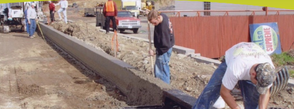
Ruhlman Brothers crew cutting a new curb
