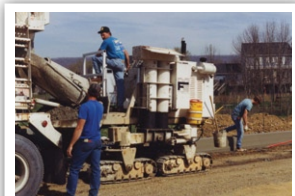
Crewmen molding a curb
